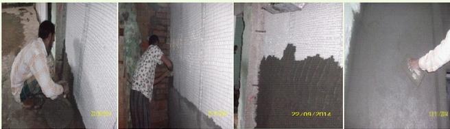
Figure 4: Initial Mortar Placing
